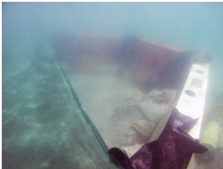
Fig. 5. The RCB cofferdam prior to the last length of shade cloth being deployed. (J. Carpenter).
