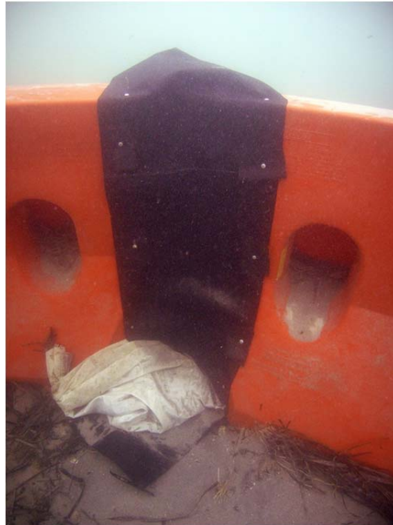
Fig. 3. Plastic tarp coursing anchored over the gaps between the RCBs with zinc tek screws. (J. Carpenter).
